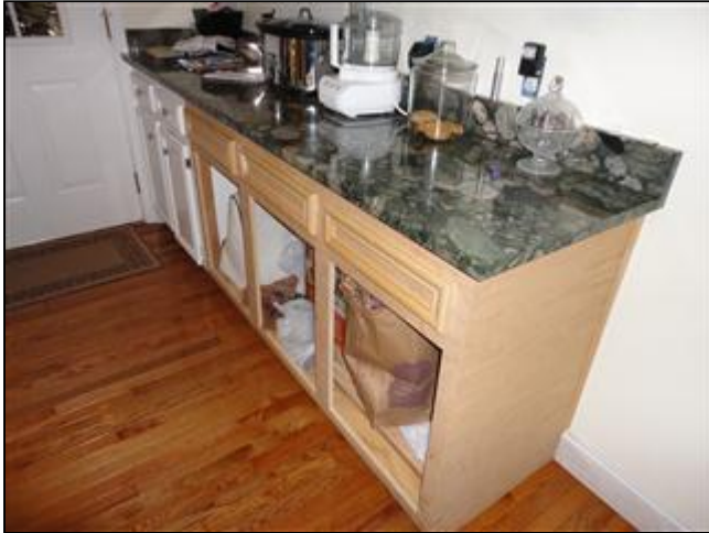
4.4 Item 1(Picture) Kitchen base cabinet missing doors
