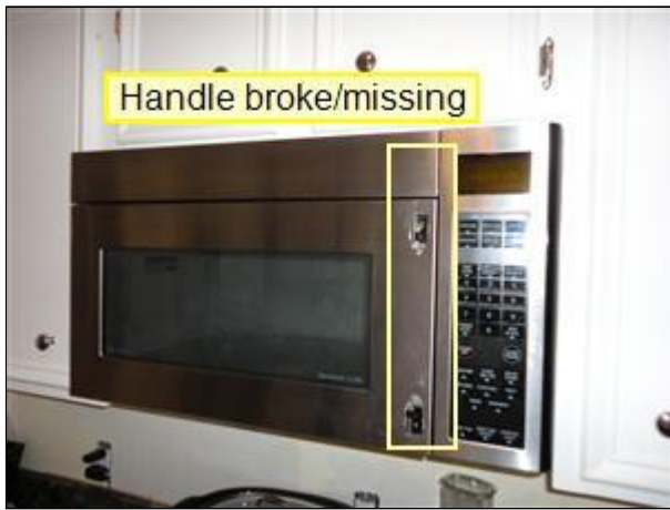
10.3 Item 1(Picture) Microwave handle missing
