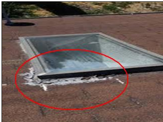
1.2 Item 1(Picture) Skylight repaired area
